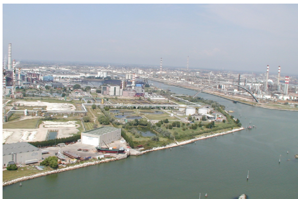
Figure 3: the industrial area of Porto Marghera and the Fusina waste water treatment plant.
