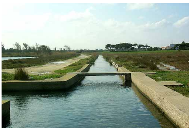
Figure 2: View of the Giammatteo canal
